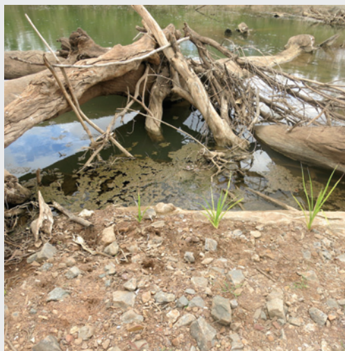
Large woody debris in the McArthur River diversion channel: providing fish habitat, protecting new revegetation, stabilising banks and reducing erosion.
