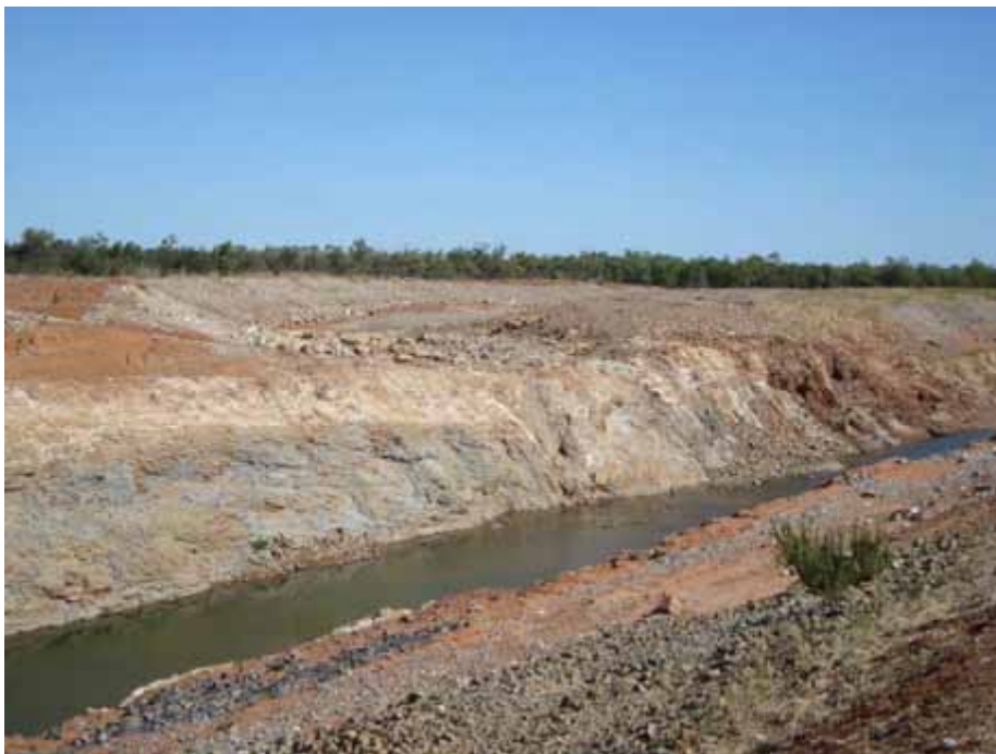
Plate 24 - McArthur River diversion, rockier section, towards upstream end (minor slumping resulting in screen pile in channel) (June 2009).
