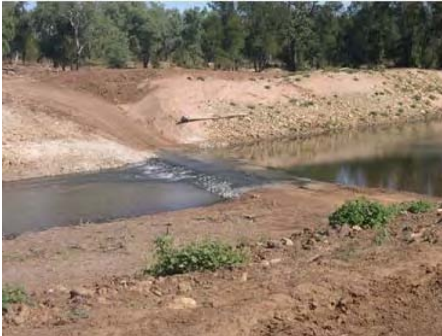
Plate 5 - McArthur River ford crossing. (Note log on bank deposited during wet season flood). (June 2009).
