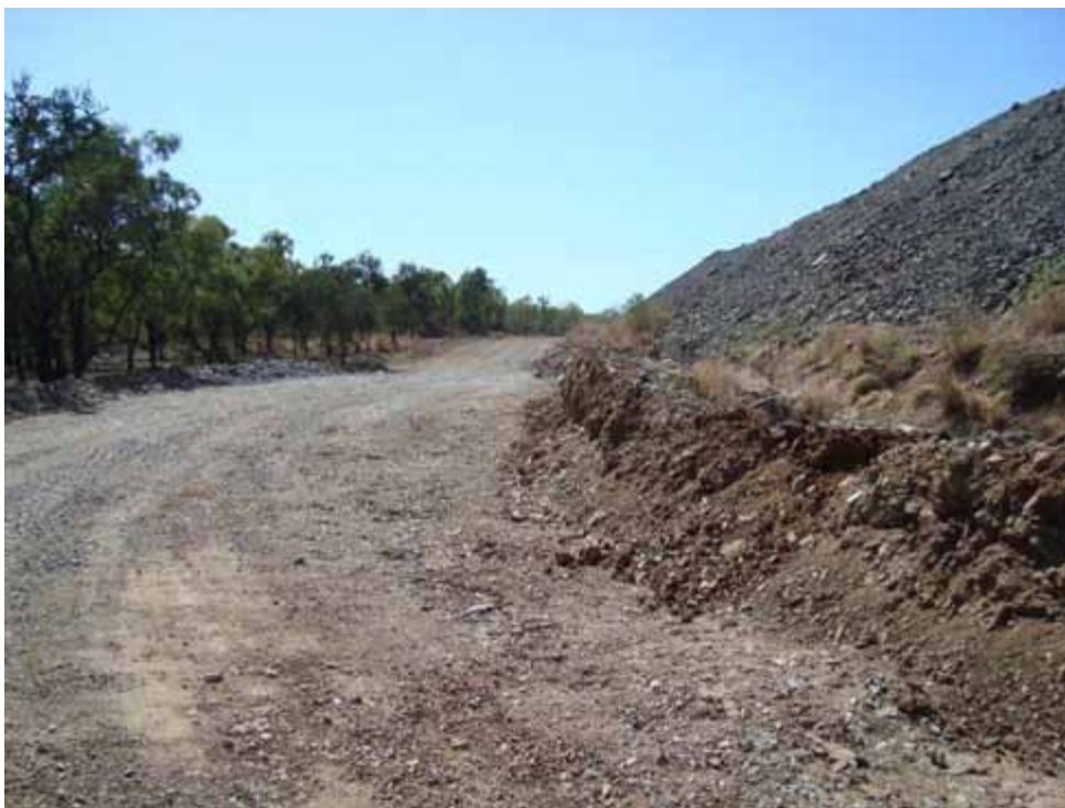
Plate 18 - Reconstructed road after washout that resulted from sump overflow (June 2009).
