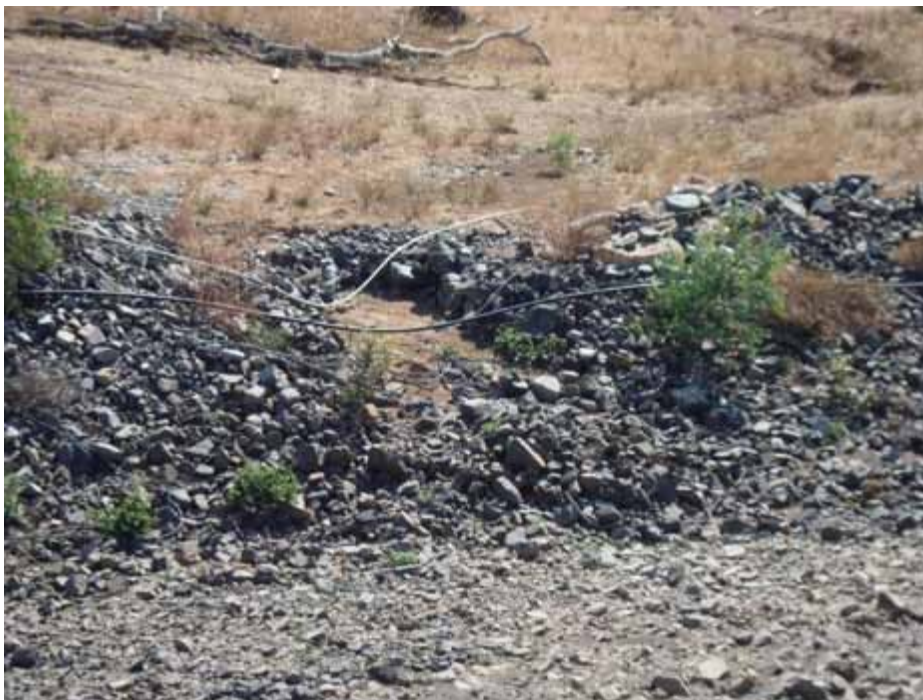
Plate 20 - Minor scour of rock armour can be seen within Barney Creek river diversion channel protection works (June 2009).
