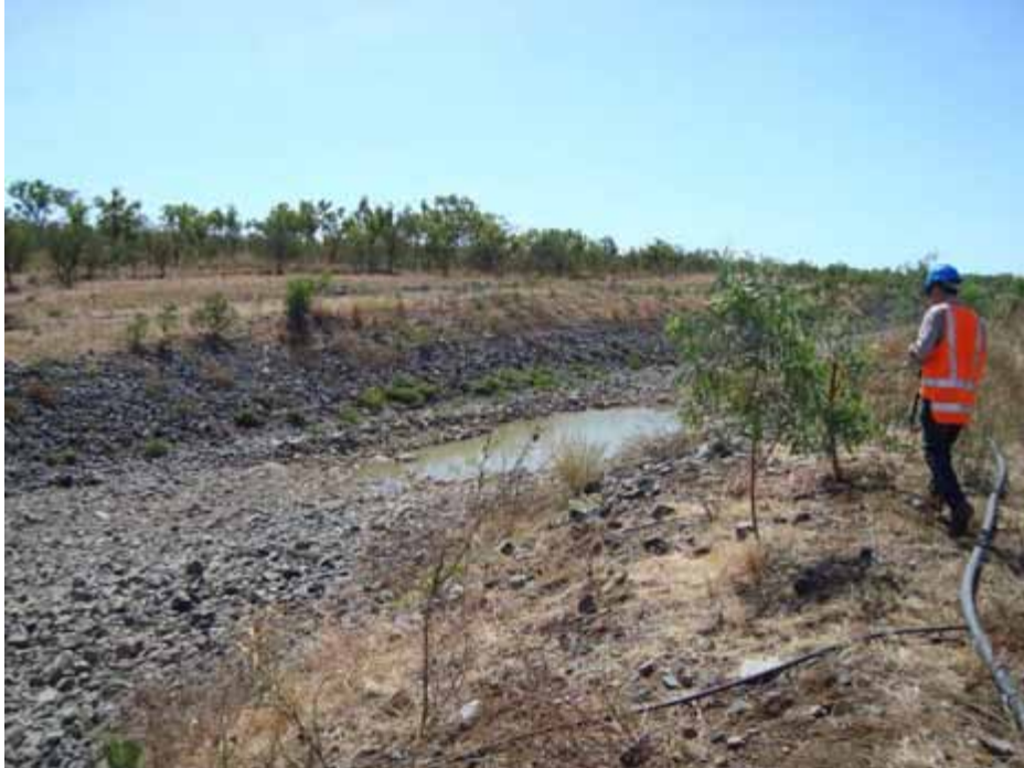
Plate 19 - Barney Creek river diversion works with rock armouring (June 2009).
