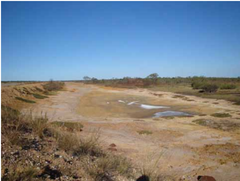
Plate 29 - Bing Bong spoil dump embankment with downstream spoon drain. Embankment deeply eroded and in disrepair. Salt crystallisation deposited from seepage can be seen on the outside of spoil wall (June 2009).
