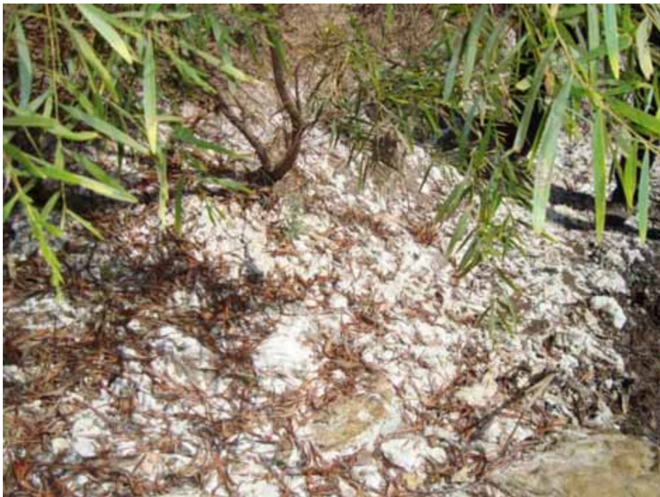
Plate 14 - Surprise Creek channel bank exhibits evidence of continued steady seepage through the presence of salt and iron below northern embankment of Cell1. Closer inspection shows that the rocks have been eroded. (June 2009).
