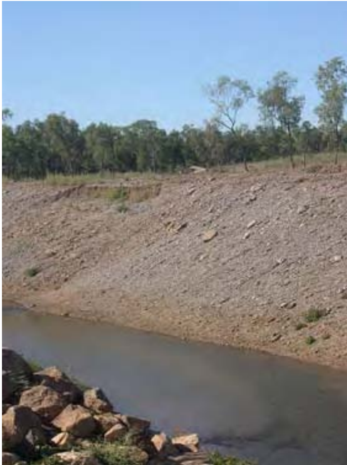
Plate 7 - McArthur River bank erosion/slumping (June 2009).
