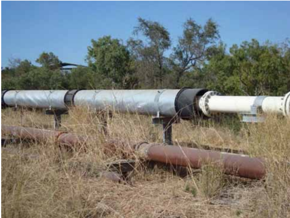
Plate 11 - TSF abutment of TSF Pipeline Bridge over Barney Creek (June 2009).
