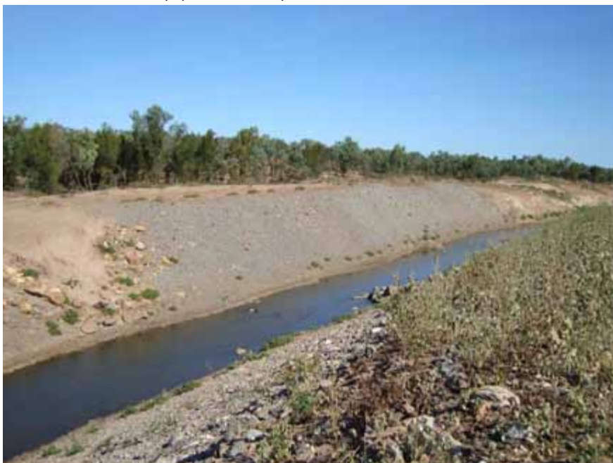
Plate 26 - McArthur River diversion, rock armour where the channel banks have a more soil profile (June 2009).
