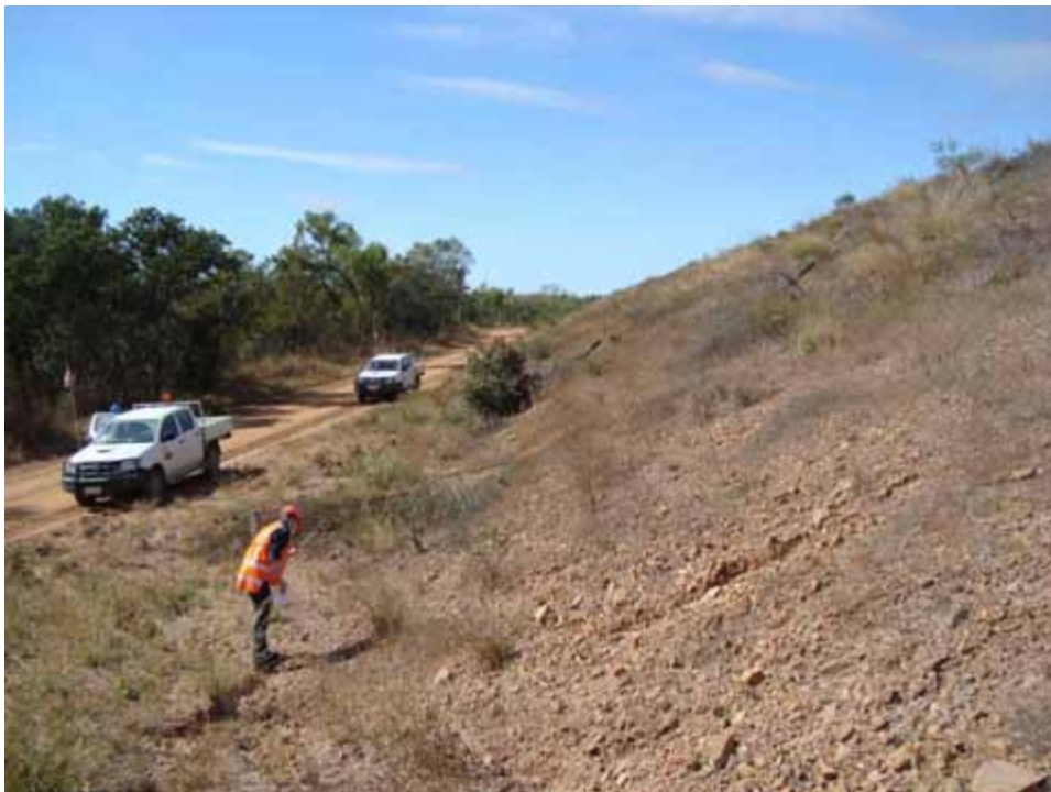
Plate 12 - Cell 1 downstream northern embankment, approximately midway along, adjacent to Surprise Creek (June 2009).
