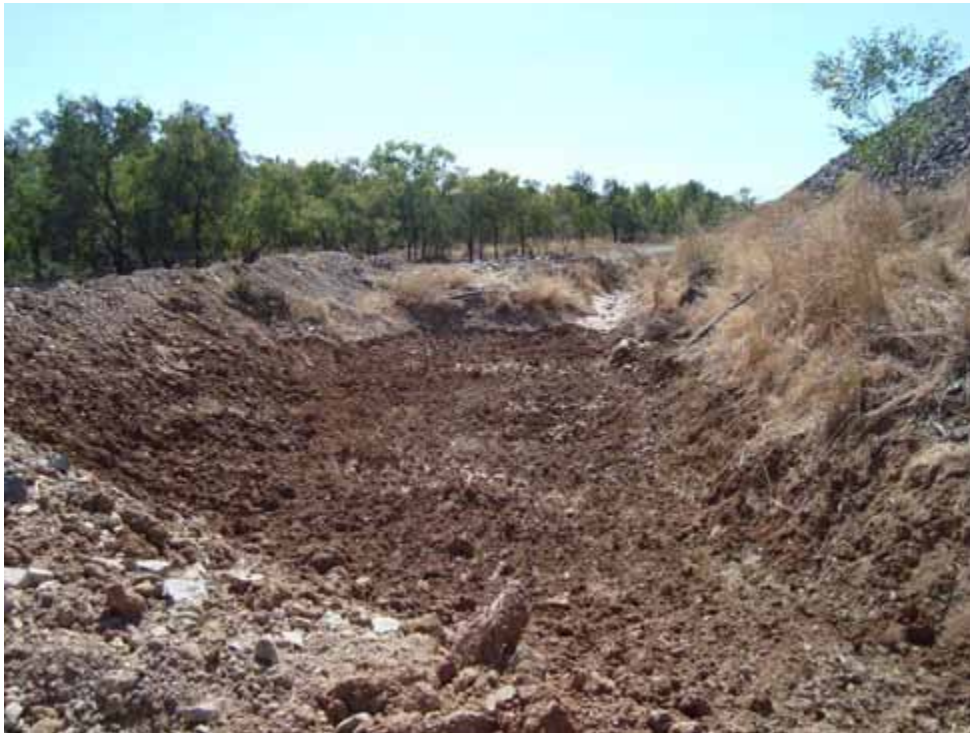
Plate 17 - MRM remediated ROM sump following overtopping during 08/09 wet season (June 2009).
