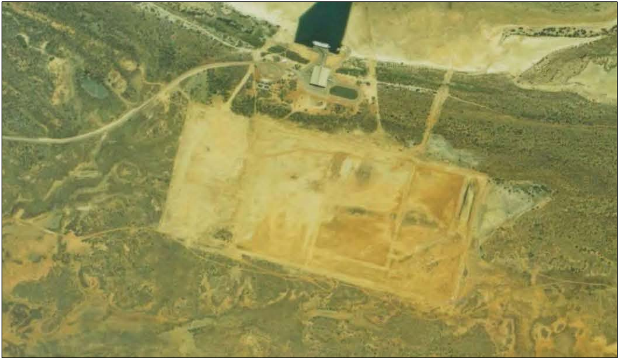
Source: Northern Territory Department of Infrastructure and Planning
