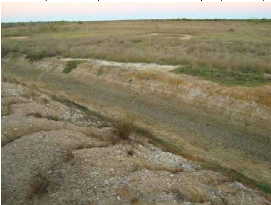
Plate 28 - Bing Bong spoil dump embankment with downstream spoon drain. Embankment deeply eroded and in disrepair (June 2009).
