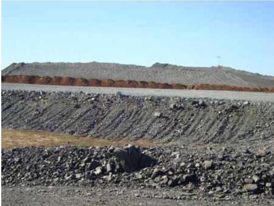
Plate 27 - Overburden Emplacement Facility cell currently under construction. Clay paddock dumped in front of current dump lift (June 2009).
