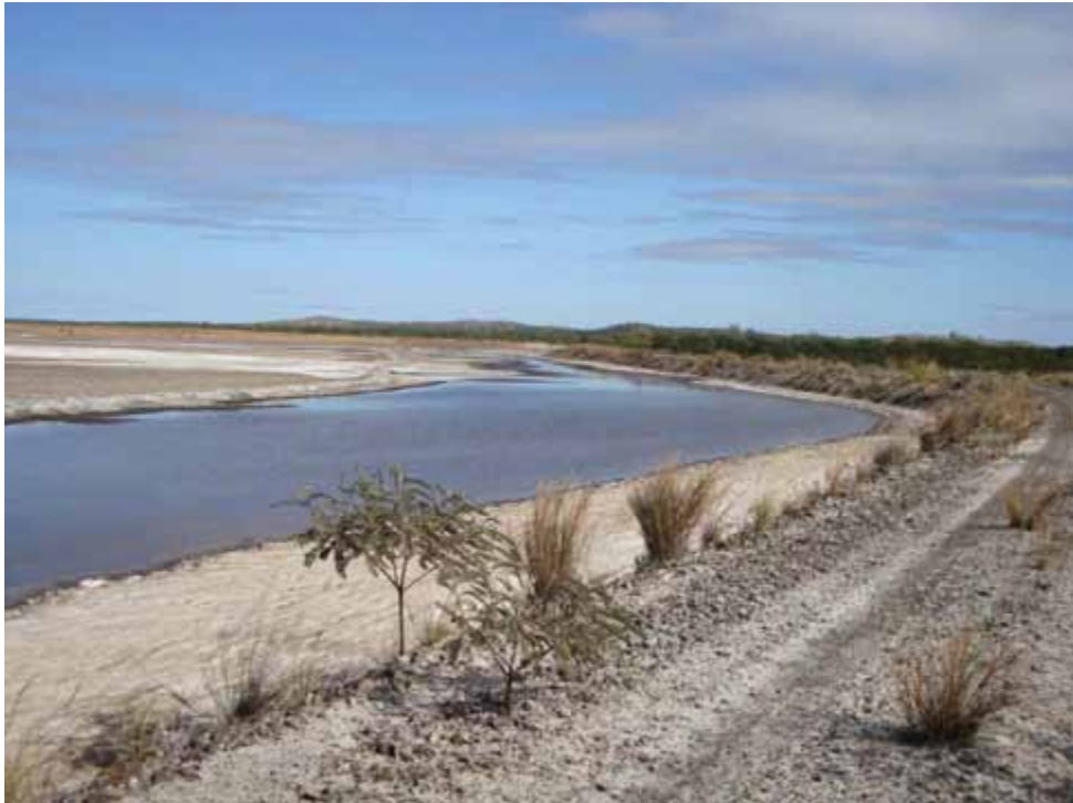
Plate 13 - TSF Cell 1 upstream northern embankment, approximately midway along. Pounded water on top of TSF (June 2009)
