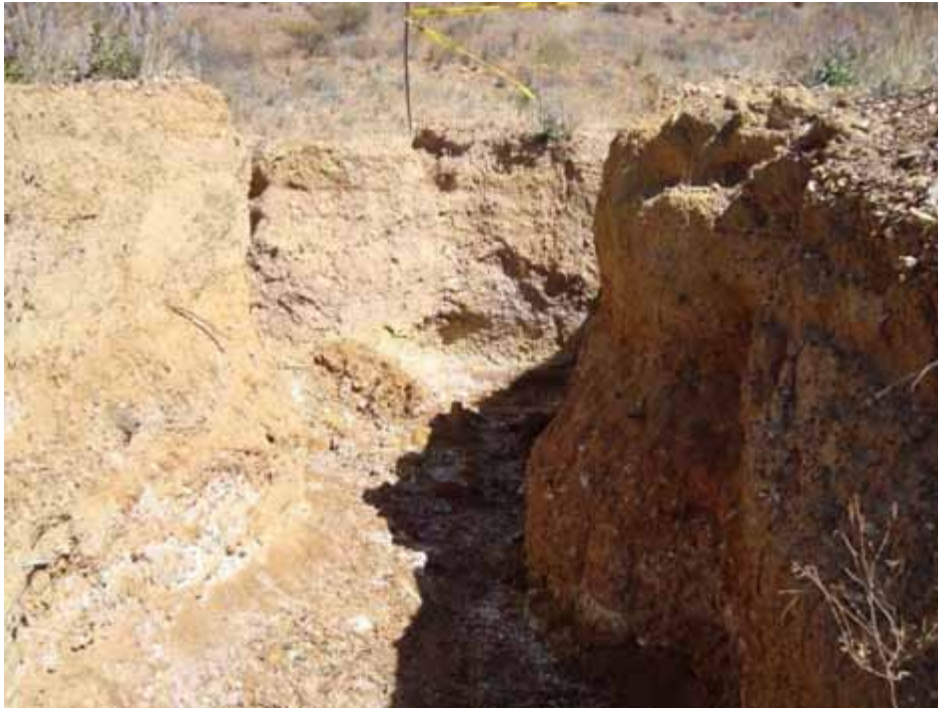
Plate 15 - Washout below TSF Cell 1 northern embankment, approximately midway along. Considerable surface expression of salt (June 2009)
