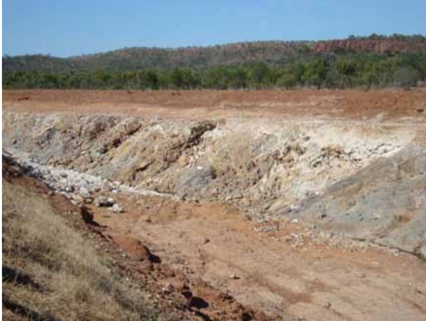
Plate 25 - McArthur River diversion, rockier section, towards upstream end (some minor wedge failures as weaker material has been washed out leaving unstable harder blocks) (June 2009).
