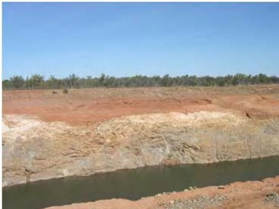
Plate 6 - McArthur River bank erosion/slumping (June 2009).
