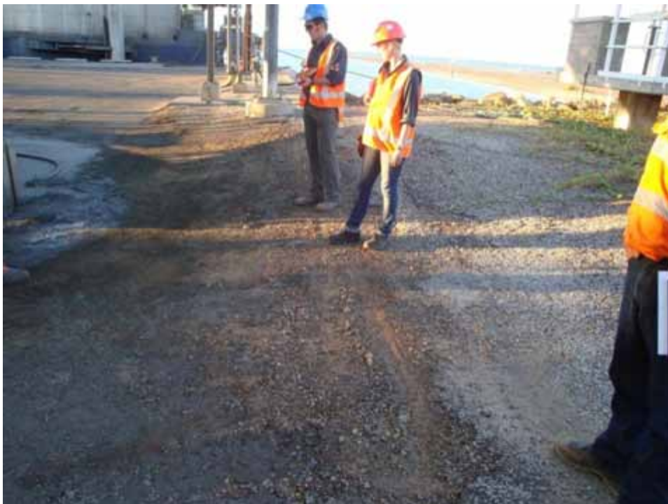
Plate 4 - Area of soil contamination beneath the Bing Bong Port load out conveyor sump/drain where bitumen had eroded expose the soil beneath (June 2009).
