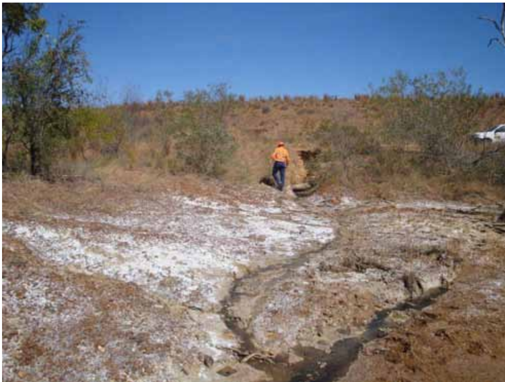
Plate 16 - Extensive surface salt downstream of second erosion gully approximately midway along northern embankment of TSF Cell 1. Seepage possibly along soil/rock interface (June 2009).
