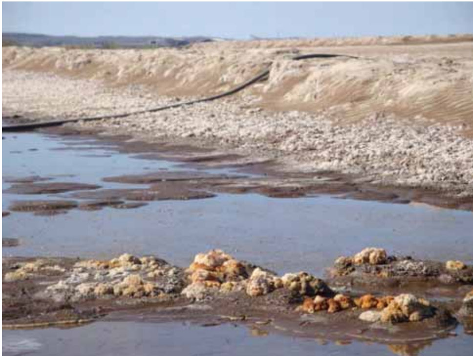
Plate 1 - Iron sulfates along beached areas of ponded water at the surface of TSF Cell 1, indicating acidic conditions (June 2009).
