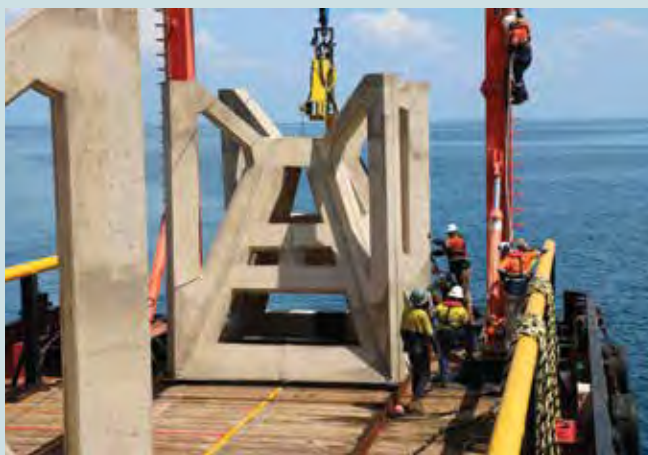
Artificial reef modules being deployed across the greater Darwin region
