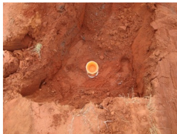
Capped at completion of hole. Dug out/cut/plugged during rehab. After rehabilitation.
