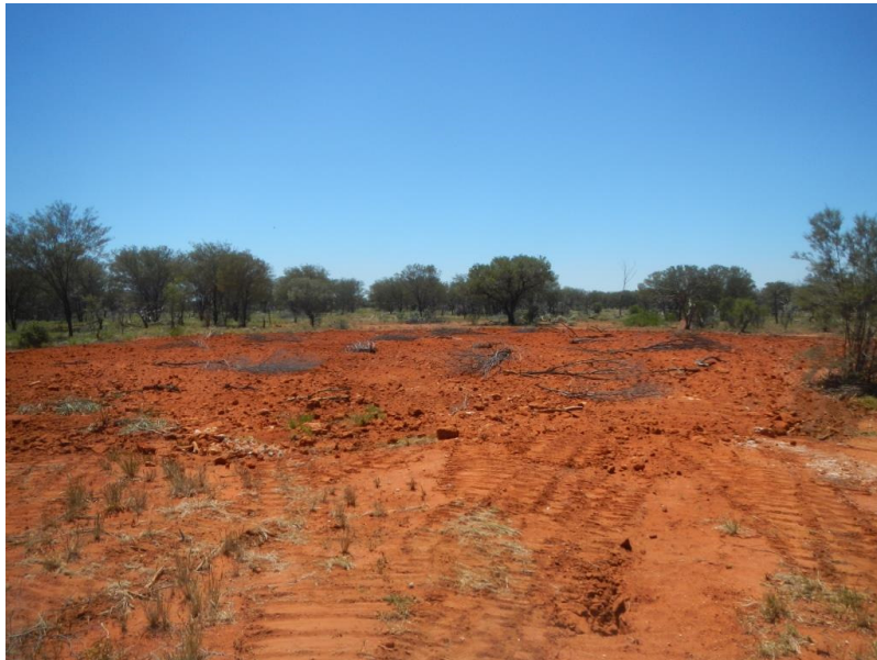
Pit 4 backfilled with topsoil re-spread on 28/10/2016
