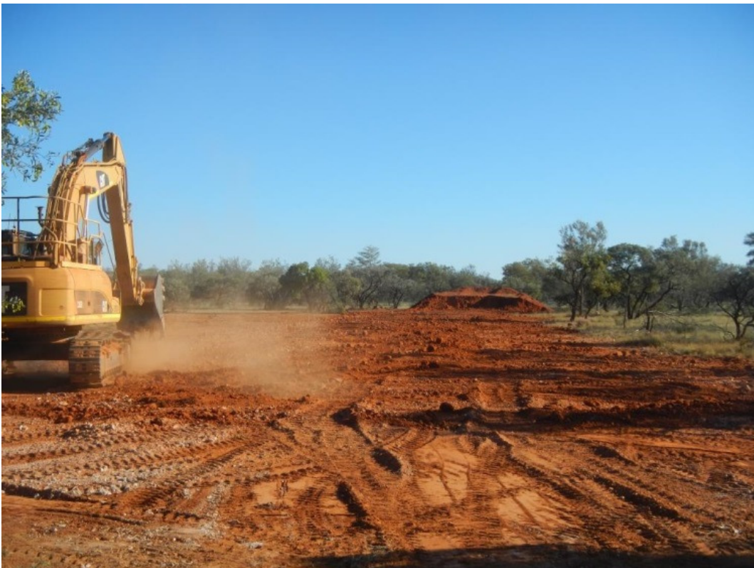
Re-spreading topsoil on BCRC138 Pit 3 on 28/10/2016
