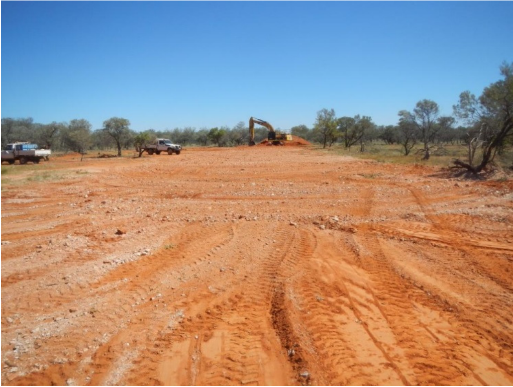
BCRC138 Pit 3 rehab in progress 28/10/2016
