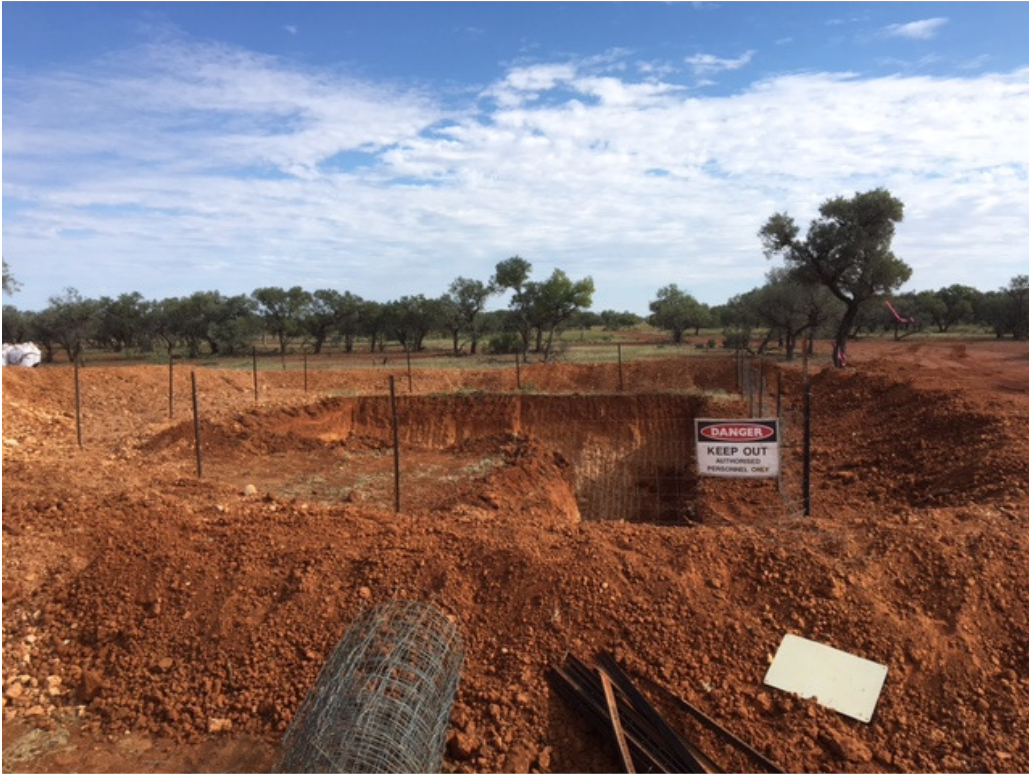
Existing Costean 5 (ARC177) which is to be deepened, sample taken and then backfilled and rehabilitated
