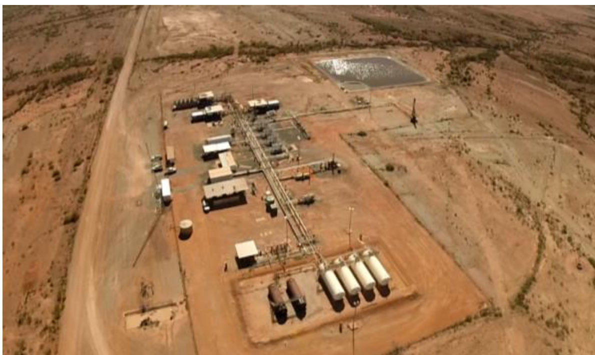
Figure 6-6: Aerial image of Mereenie Eastern Satellite Station
