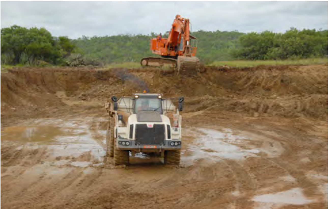
Reshaping of waste rock dump at Mount Todd
