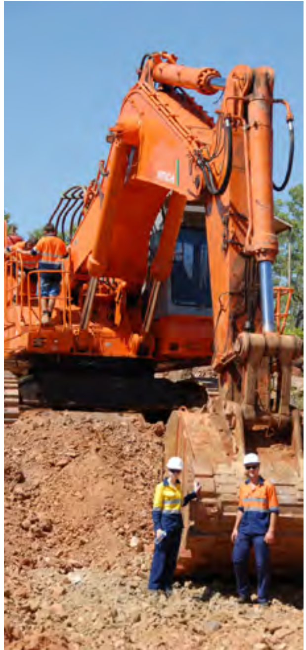
Excavation of a diversion drain at Mount Todd
