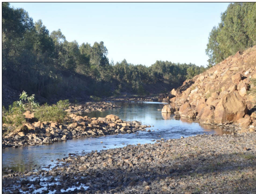
Plate 3 – Barney/Surprise Creek Confluence During IM Visit, May 2012
