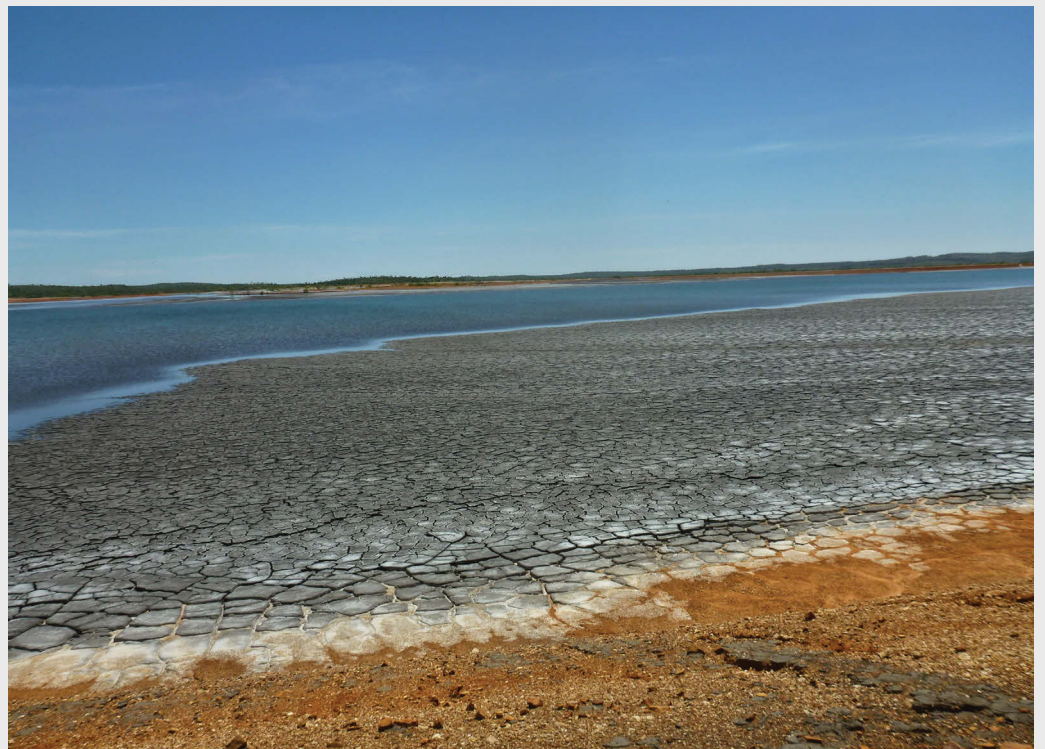
TSF Cell 2, showing the tailings beach
