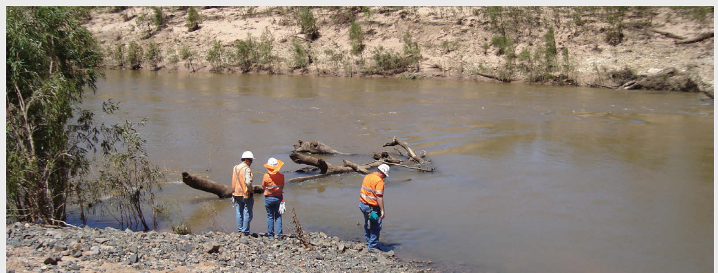
Part of the McArthur River diversion channel, March 2014
