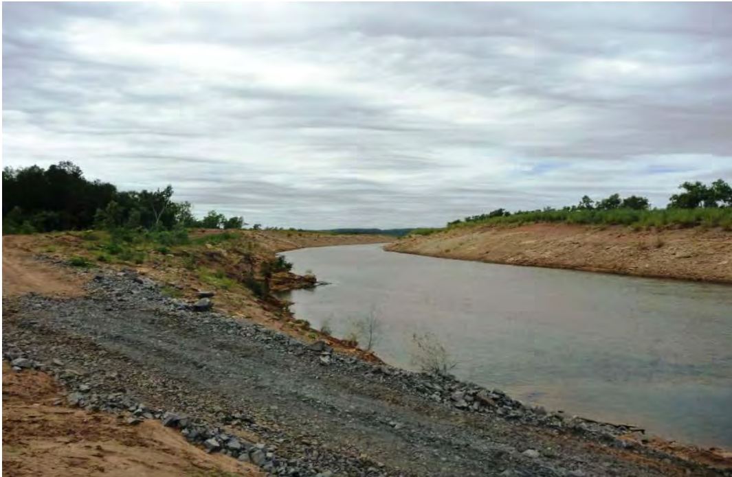
Plate 32 - Looking downstream along the McArthur River diversion channel from the ford.
