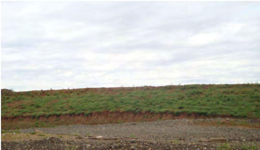
Plate 31 - Scour at the toe of the main Mine levee due to overland flows of the McArthur River during 2009/2010 wet season flooding – (see section 8.8.5)
