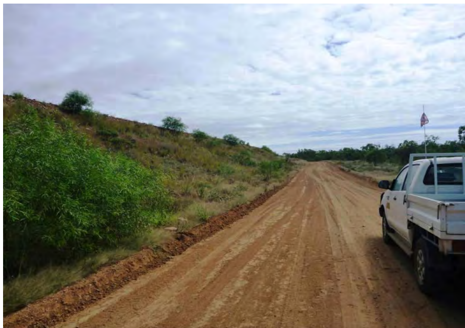
Plate 20 - TSF Cell 1, Northern embankment looking west
