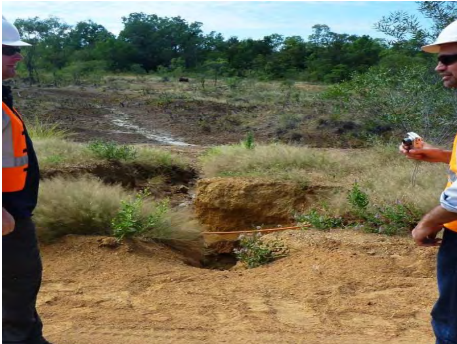
Plate 18 - Evidence of piping erosion on the northern track edge of TSF Cell 1.
