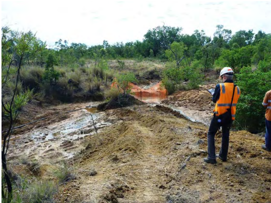
Plate 17 - Seepage expressing into Surprise Creek, northern boundary of TSF Cell 1
