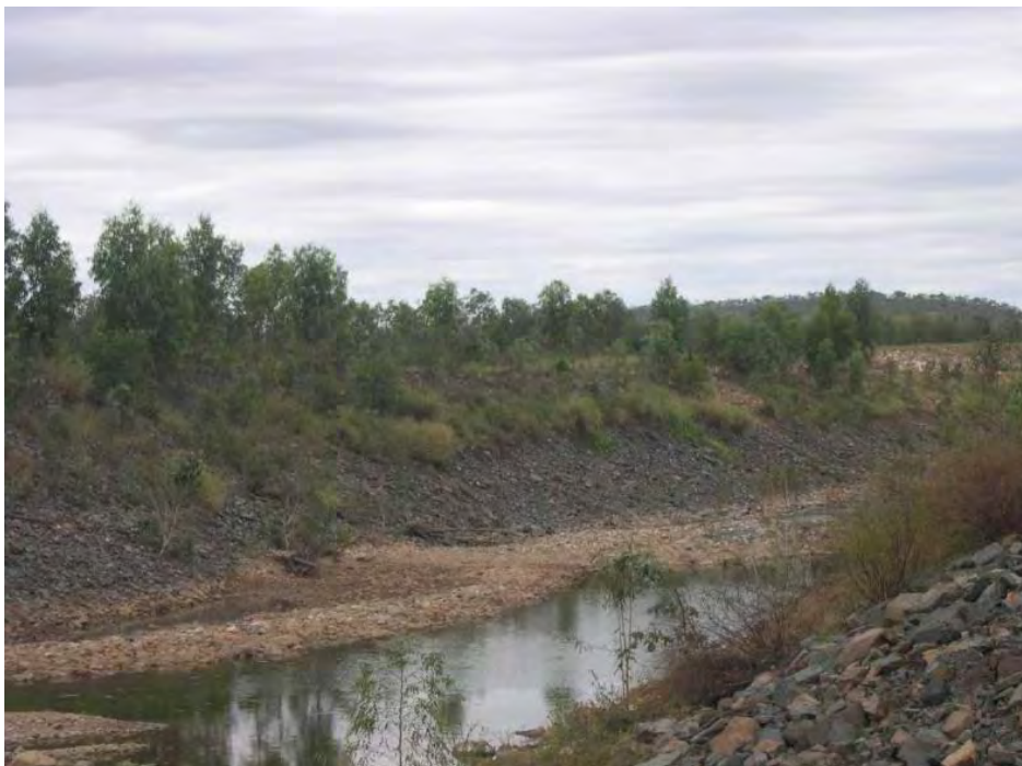
Plate 48 - Barney Creek channel, just downstream of the Surprise Creek confluence.
