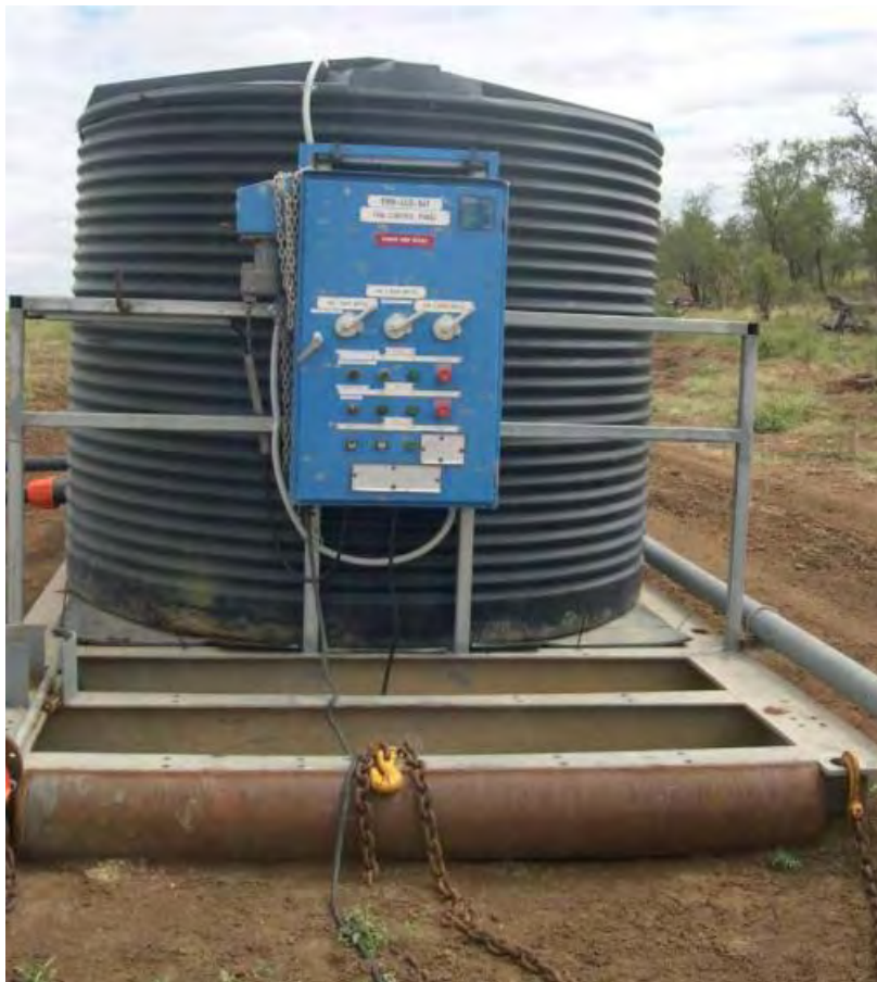
Plate 45 - The new irrigation sled structure which is now used for the irrigation of the river diversion channel rehabilitation works
