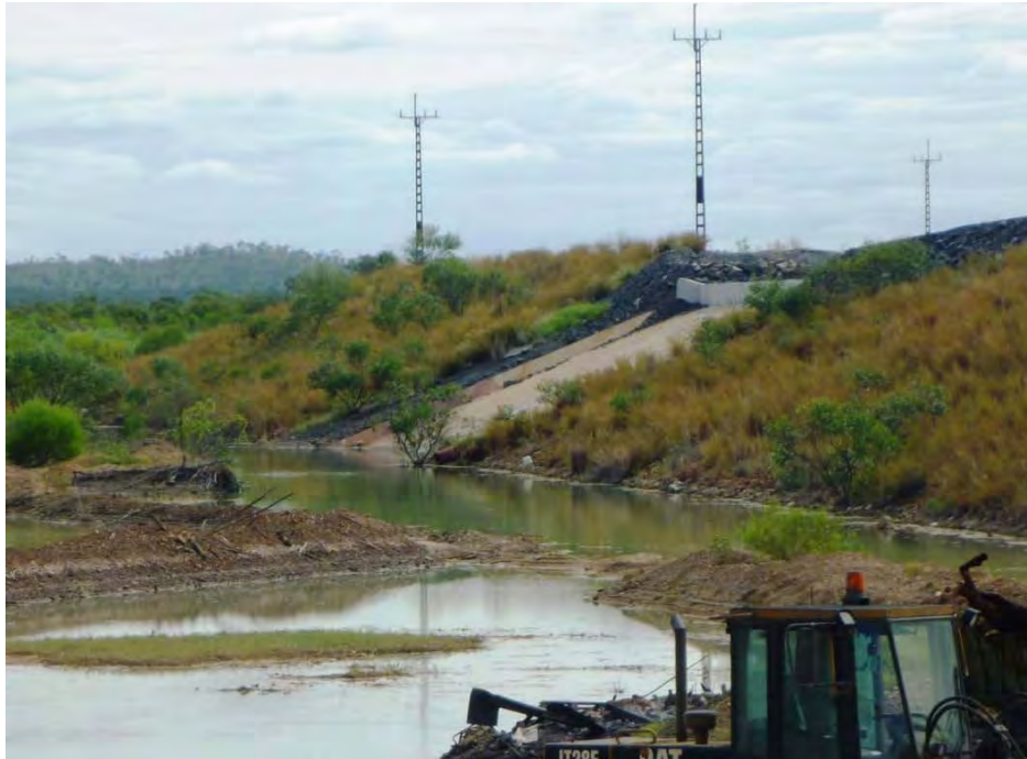
Plate 25 - TSF Cell 2 Spillway. Seepage evident through concrete spillway.
