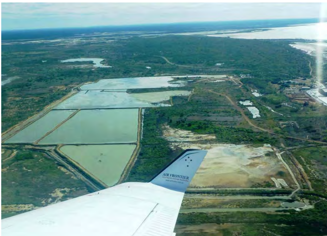
Plate 27 - Bing Bong Spoil Dump – Aerial view looking west.
