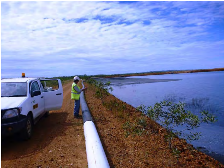
Plate 23 - TSF Cell 2 Western Embankment, showing tailings pipeline and Standing Water against embankment of Cell2.
