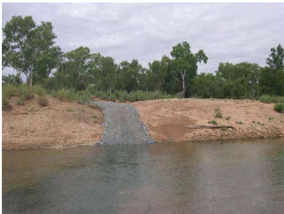
Plate 43 - View of ford (under water), looking east across the river diversion channel (May 2010).
