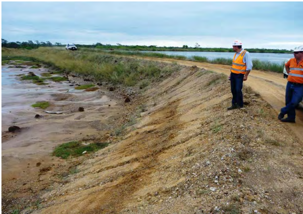
Plate 28 - Bing Bong Spoil Dump. Repaired Section of embankment. Seepage visible on left.
