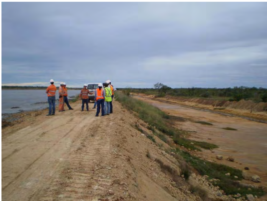
Plate 2 - Remediated Bing Bong Dredge Spoil Pond wall (centre) with newly-constructed outer spoon drain (right) and recently deposited dredge material (Left).
