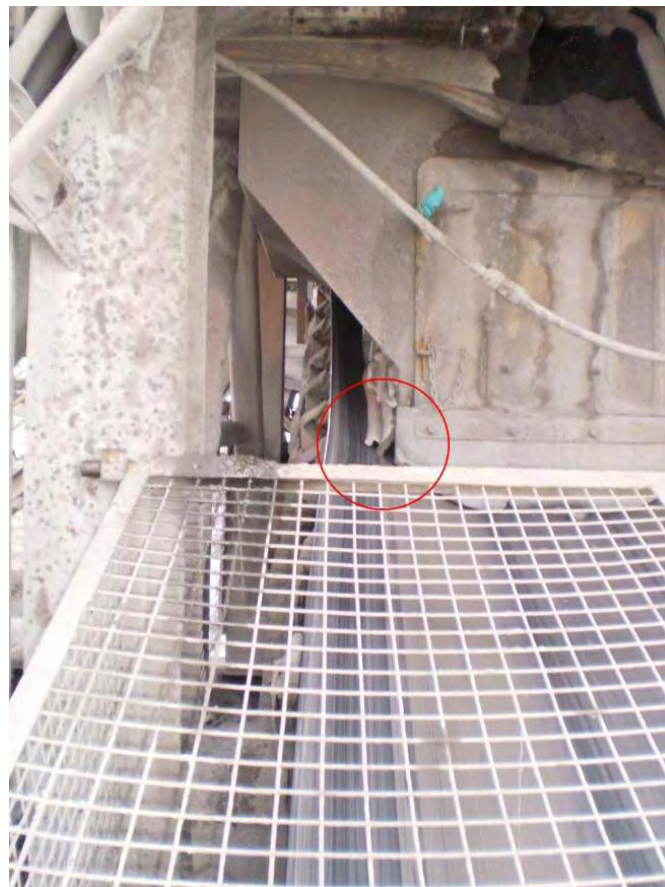
Plate 5 - Pacrim conveyor with double-lipped lining (circled) to aid dust suppression.
