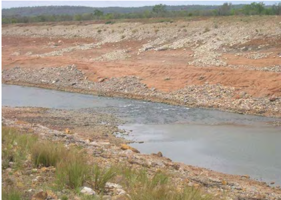
Plate 44 - View of one of the riffle zones in the McArthur River diversion channel
