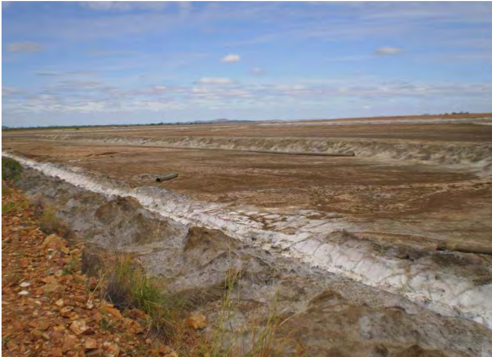
Plate 4 - TSF Cell 1 with incomplete clay capping.
