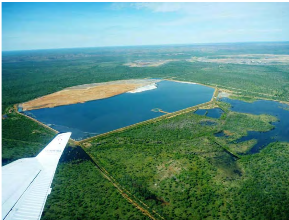
Plate 26 - Standing water very evident within TSF Cell 2. Ponded water near toe of embankment (at wing tip) is a cause for concern
