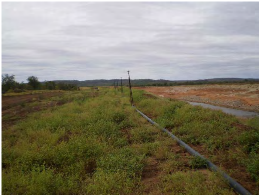
Plate 9 - New Irrigation system at the upstream section of the McArthur River diversion.
