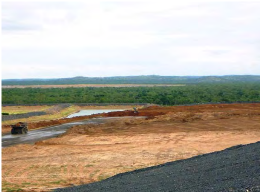
Plate 16 - Facing north-west towards the clay liner being placed for the Overburden Emplacement Facility.
