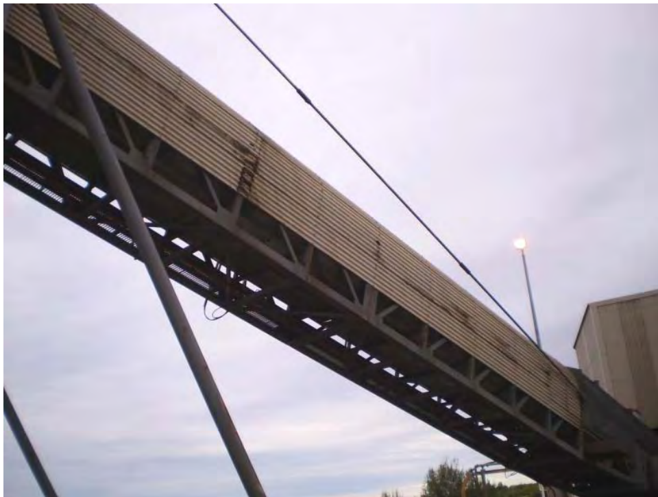
Plate 7 - Enclosed load-out conveyor at Bing Bong Port.
