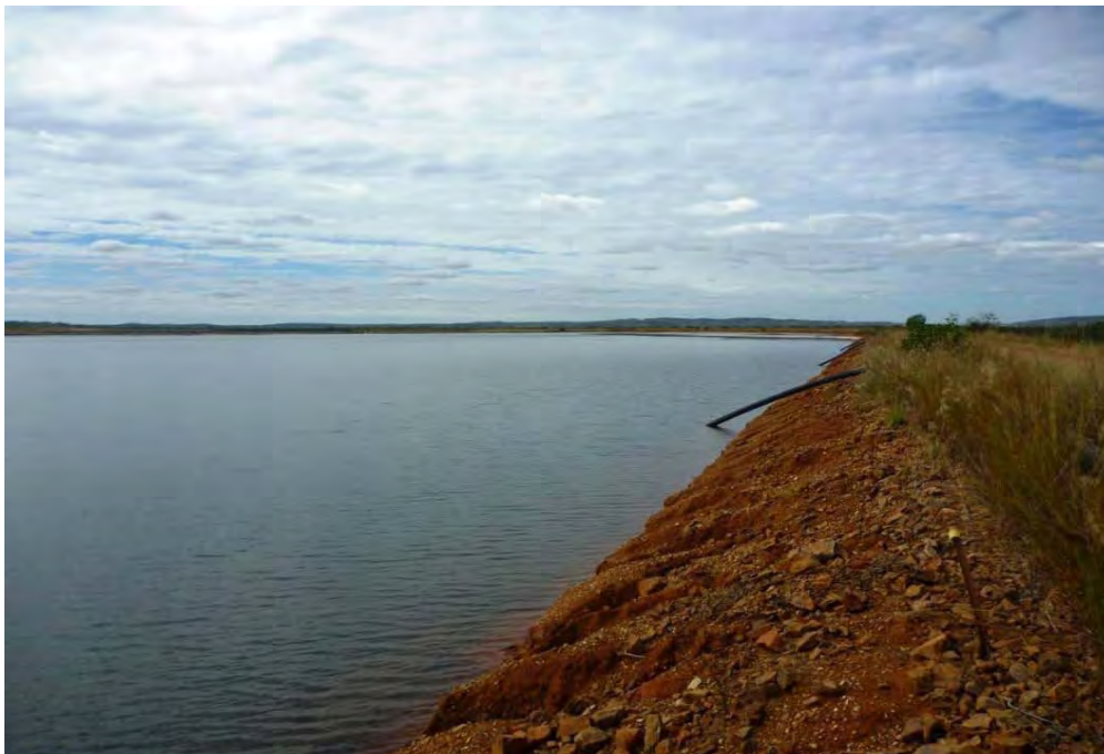
Plate 24 - TSF Cell 2: Deep body of standing water against the embankment with some erosion of the embankment occurring
