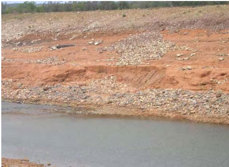
Plate 37 - Relatively minor bank erosion in the McArthur River diversion channel.
