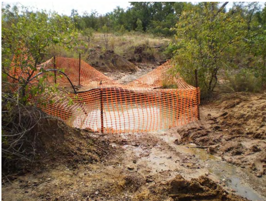
Plate 1 - Sump installed between Tailings Storage Facility Cell1 and Surprise Creek to collect leachate.
