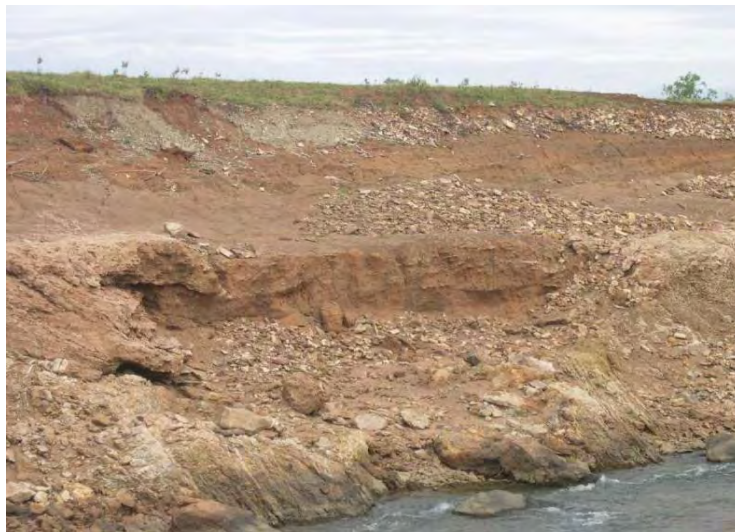
Plate 38 - An example of relatively minor bank erosion in the McArthur River diversion channel.
