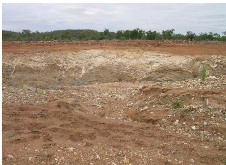
Plate 39 - Local (foreground) erosion at the top of the McArthur River diversion channel bank.
