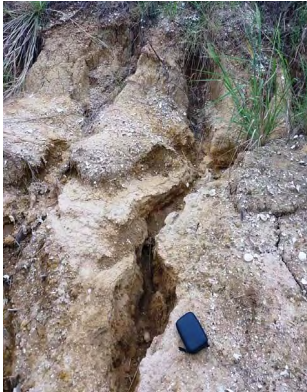
Plate 30 - Bing Bong Spoil Dump. Piping erosion in Eastern embankment
