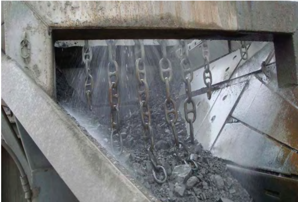
Plate 6 - Water sprays applied to ore within crushing machinery for dust suppression.
