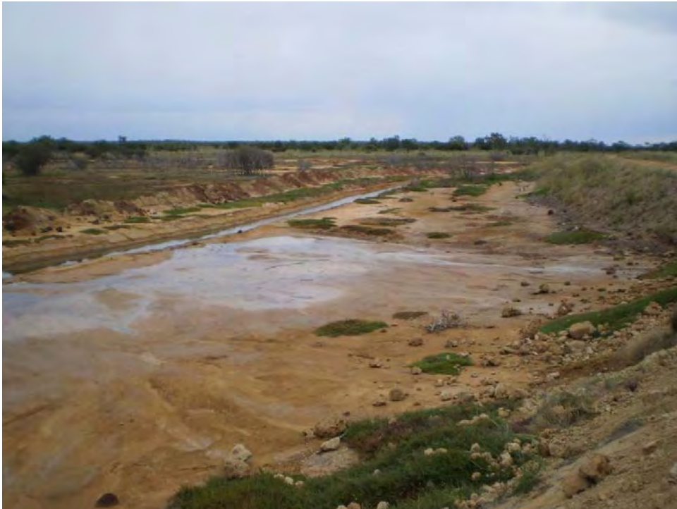
Plate 3 - Saline leachate seeping from Bing Bong Spoil pond wall towards the spoon drain.
