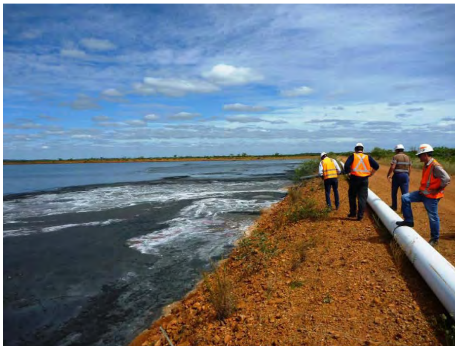
Plate 22 - TSF Cell 2 western embankment with tailings beach formed against embankment.
