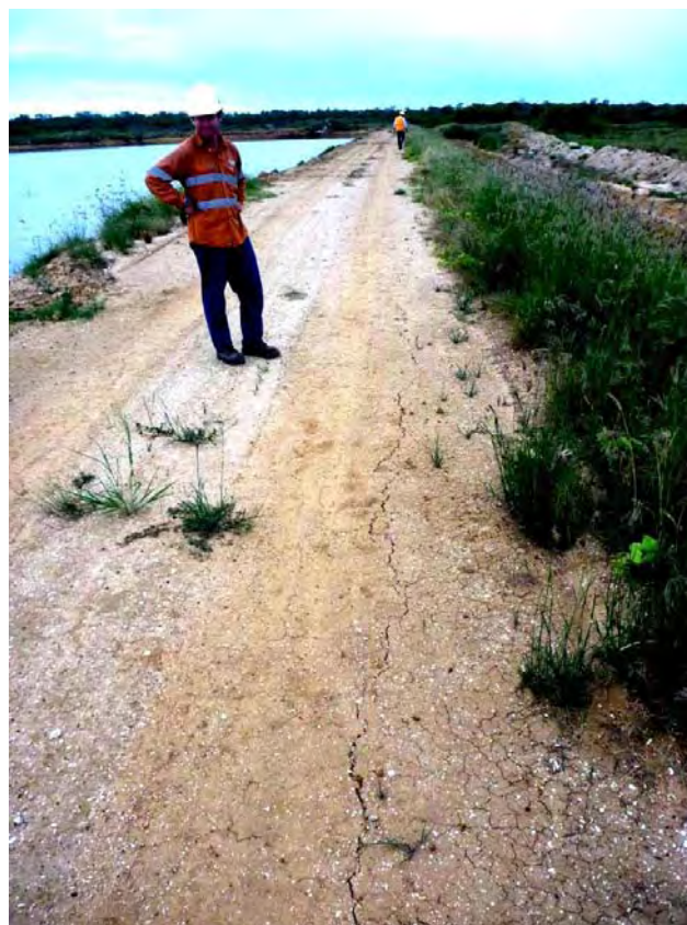
Plate 29 - Bing Bong Spoil Dump. Longitudinal cracking in Eastern Embankment
