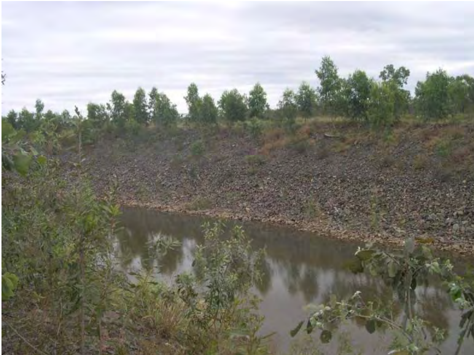
Plate 47 - As reported in the previous Independent Monitor audit report (2009) the paucity of vegetation established on the lower parts of the Barney Creek batter slope (here located just upstream of the Surprise Creek confluence) is clearly evident.
