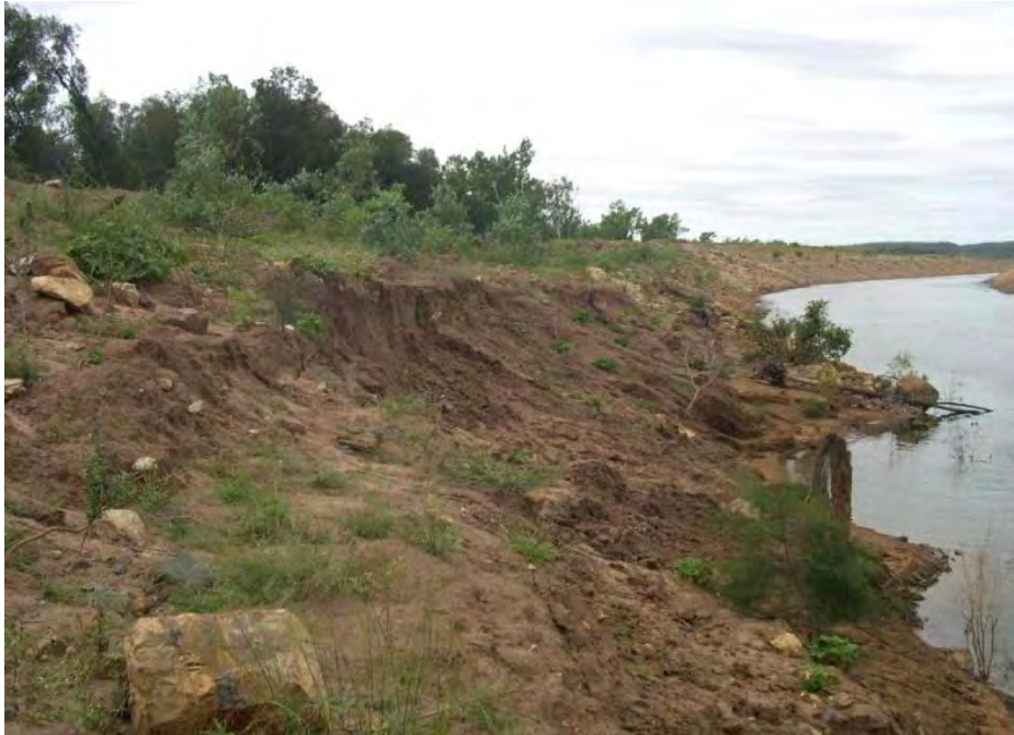
Plate 36 - Example of relatively minor bank erosion in the McArthur River diversion channel.
