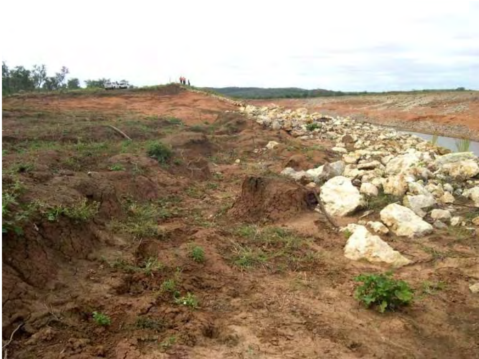
Plate 41 - View of ground conditions at the point where the flowpath from the remnant river channel empties into the diversion channel. There is clear evidence of substantial and broad erosion.
