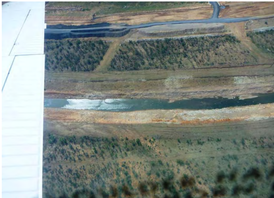
Plate 34 - View of McArthur River diversion channel from the air.
