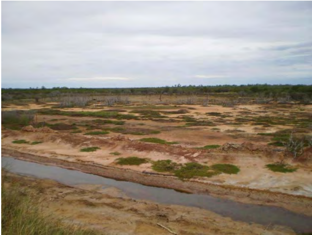
Plate 13 - Outer spoon drain at the Bing Bong Dredge Spoil to direct saline seepage from the spoil ponds to the sea.
